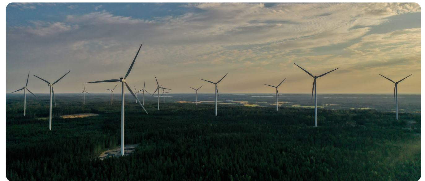
| Turbines generate clean electricity at a utility-scale Amazon wind farm.
