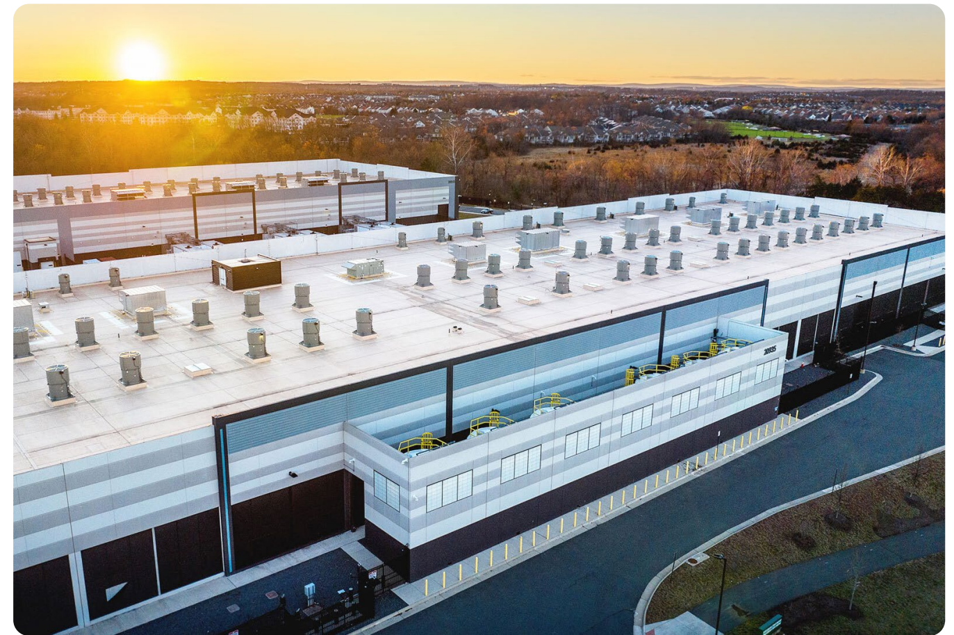
An AWS data center in Northern Virginia.
