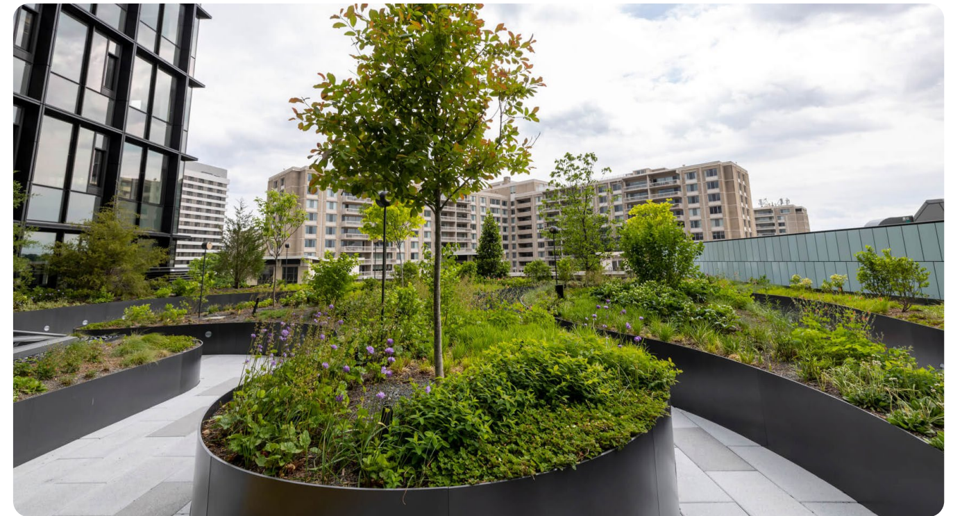
The terrace gardens at our headquarters in Arlington, Virginia, feature recycled greywater systems for irrigation.
